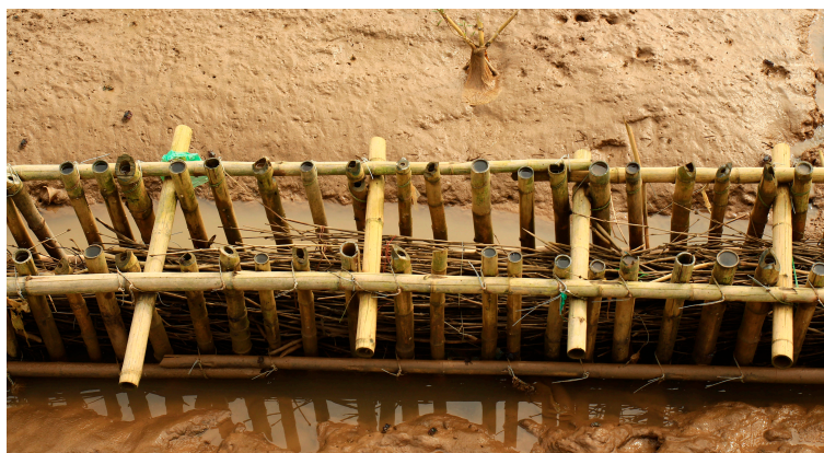
Figure 1. Wooden fences in the field [6]. The construction includes the frame (two rows of 6–8 cm diameter bamboo poles) and the inner part (a bunch of branches of 1–2 cm diameter bamboo reeds). Reproduced with permission from Dao et al. (2018), Journal of Coastal Research ; published by BioOne, 2018.
